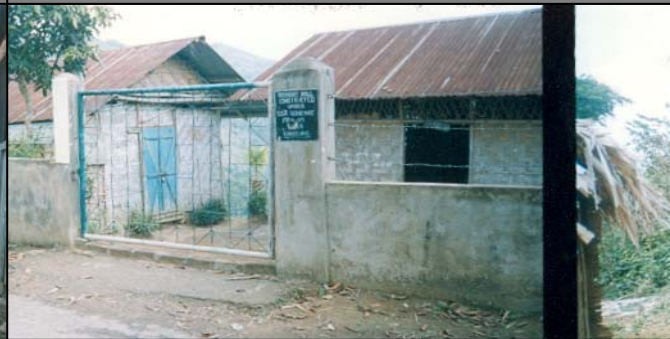
Boundary wall constructed under SSA at Kangching village
