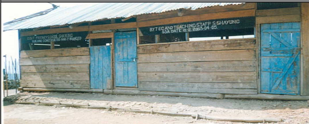
Structure constructed under SSA at Shayung village
