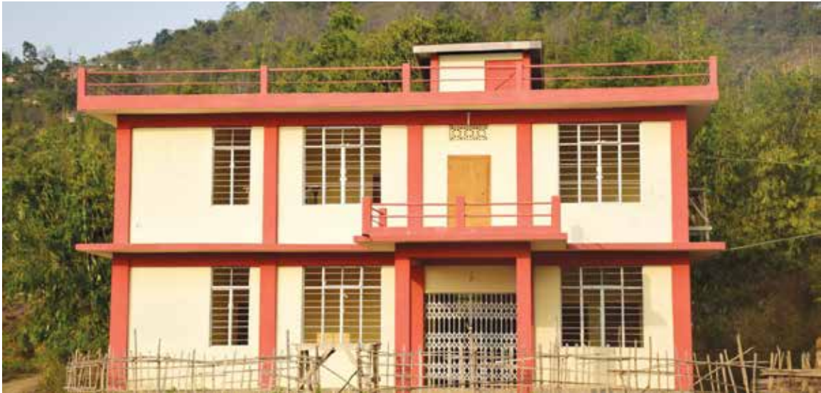
District Evaluation Office Building, Longleng.
