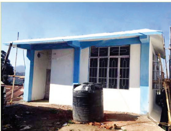
Construction of District Evaluation Office Building, Tuensang
