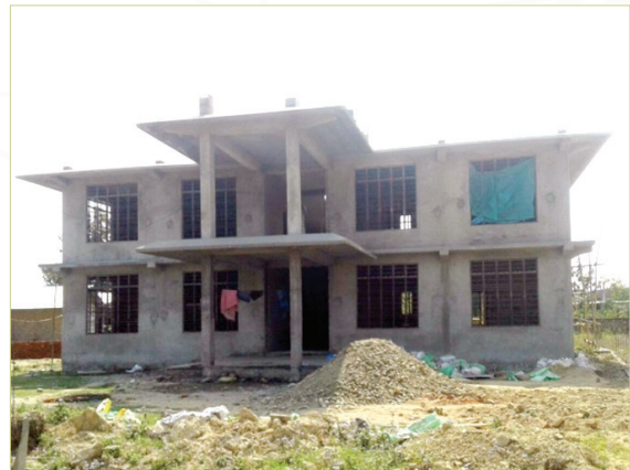
Construction of Flat type Staff Quarter at Dimapur
