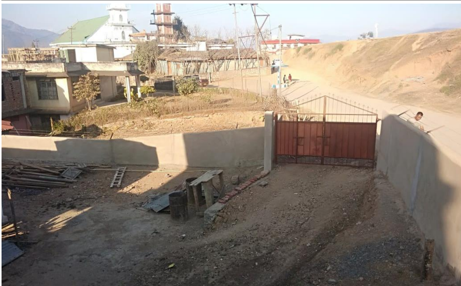
Construction of security fencing with steel gate and retaining wall at DEO Kiphire
